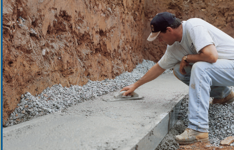
Form-A-Drain is both the footing form and the foundation drainage system, allowing you to accomplish two jobs at the same time — saving time...and money.
